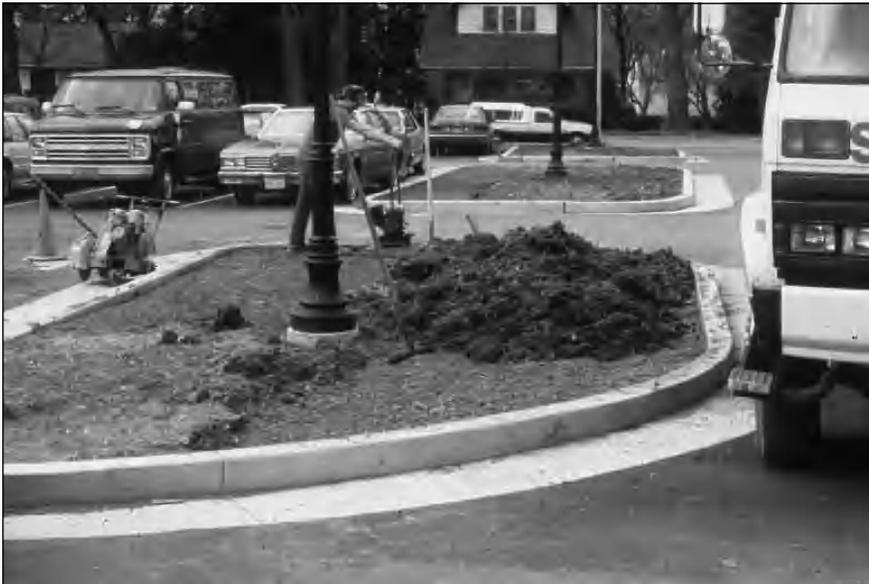
***Do not cover cement and other debris with a few inches of topsoil. All garbage and construction gravel should have been removed from these parking lot and other planting cutouts. These and other planters should be filled with topsoil or a professionally designed soil.***
